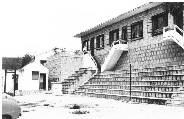
There was already a library on the Pok Oi Chuen campus.
